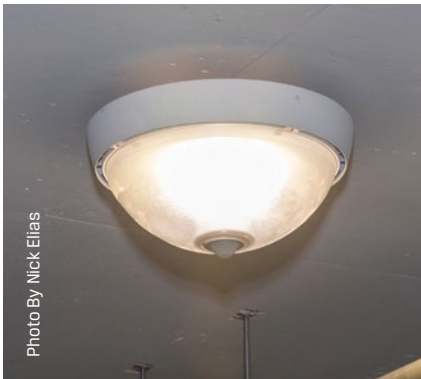
Sprig Electric installed LED lighting with motion sensors on every fixture throughout the two-level underground parking garage.
