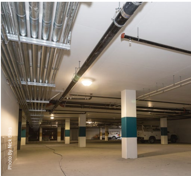
Sprig Electric installed LED lighting with motion sensors on every fixture throughout the two-level underground parking garage.
