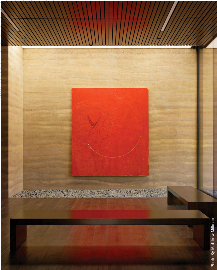
The building combines the minimalism of rammed earth and wood siding walls, with the lighter elements of aluminum and glass.
