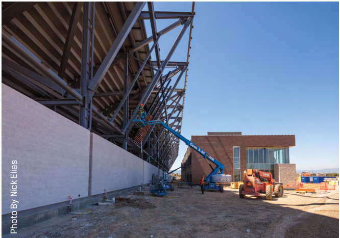
One of the biggest challenges during the initial stages of wiring the stadium was hoisting Sprig's electricians high into the air inside the structure so that lighting could be installed on the perimeter.
