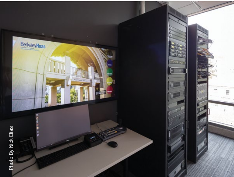
ICS wired the event control room, which enables the AV system and facilitates the transfer of content to any other lecture space within the building.
