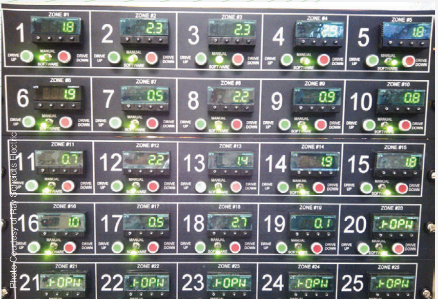
The front of the Variac Heat Flux Control Panel built and installed by Ray Scheidts Electric.
