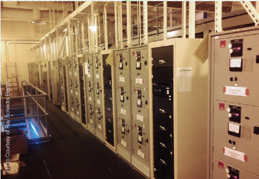
690 Variac cabinets installed by Ray Scheidts Electric next to the space simulation chamber.
