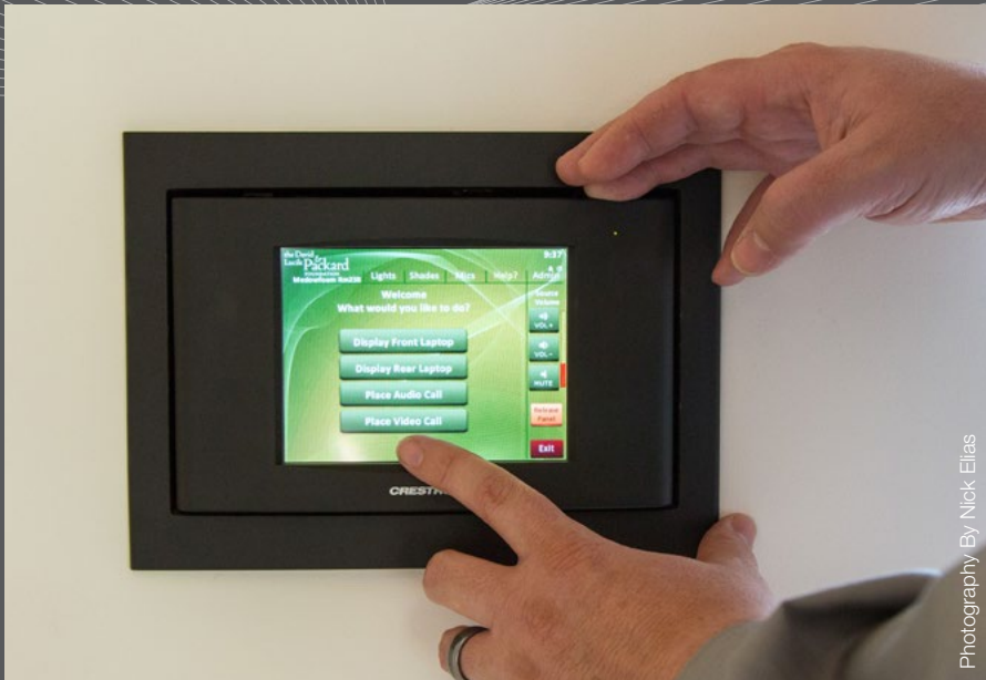
ICS wired the flat panel display that controls multi-functions in each conference room, including screens, shades and lights.
