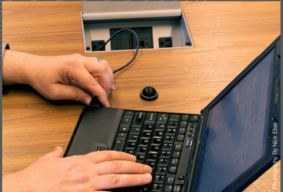
ICS wired HDMI input on conference room tables so a laptop can be connected to display content on a flat screen or projector screen.
