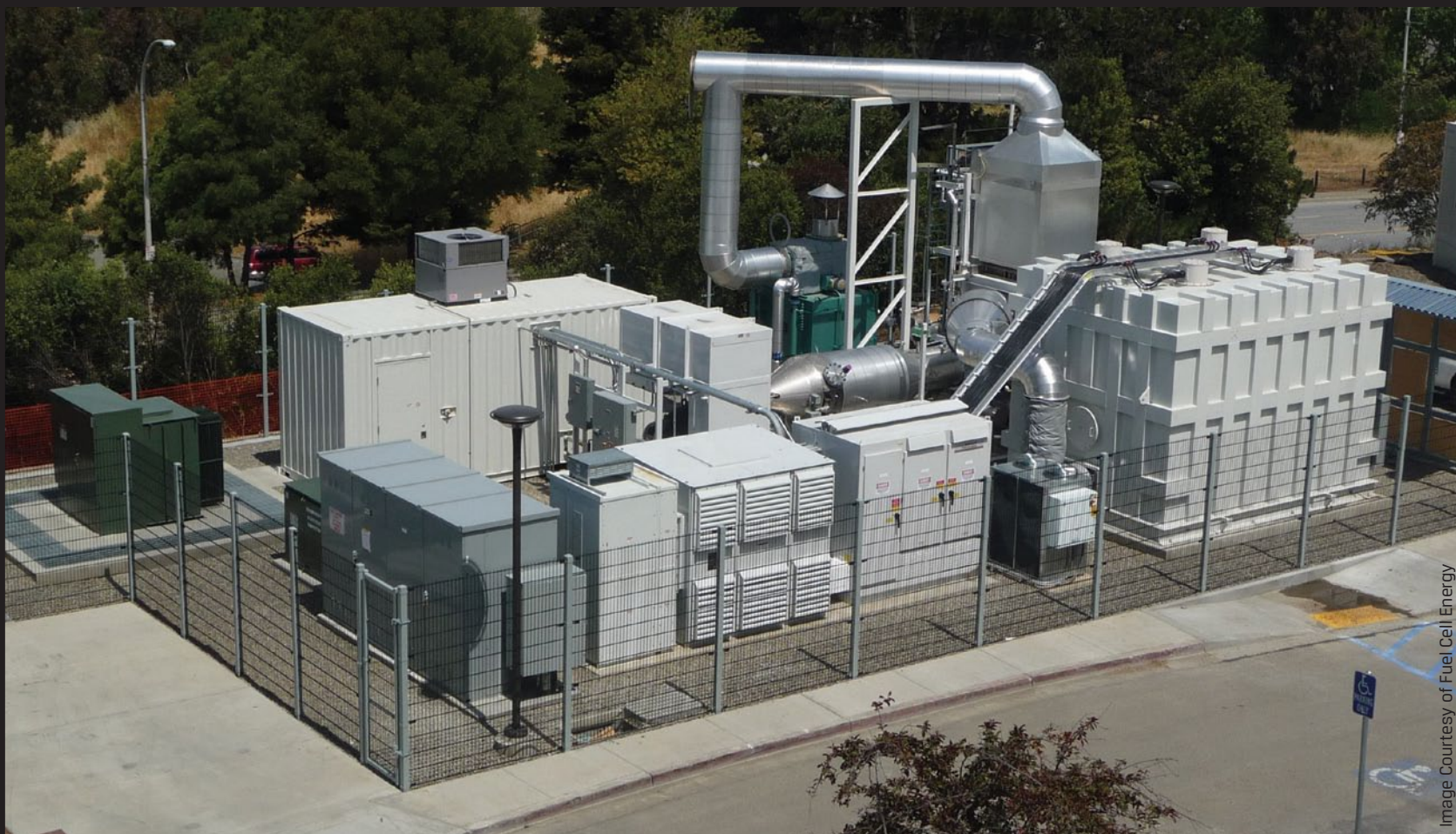
A 1.4 megawatt DFC1500 fuel cell by Fuel Cell Energy like the one installed by Sprig Electric at San Francisco State University.
