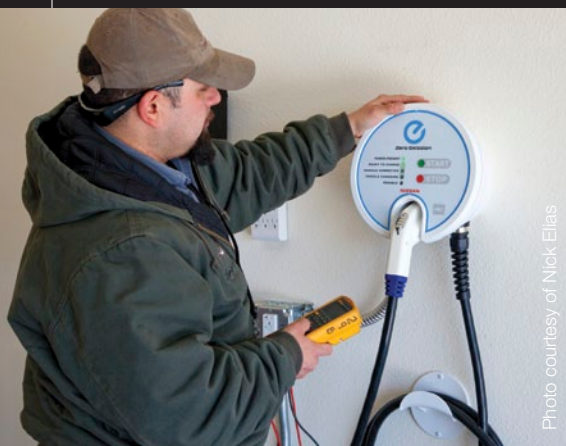
IBEW Local 332 Installer Paul Pulido installs a Residential Electric Car Charger.
