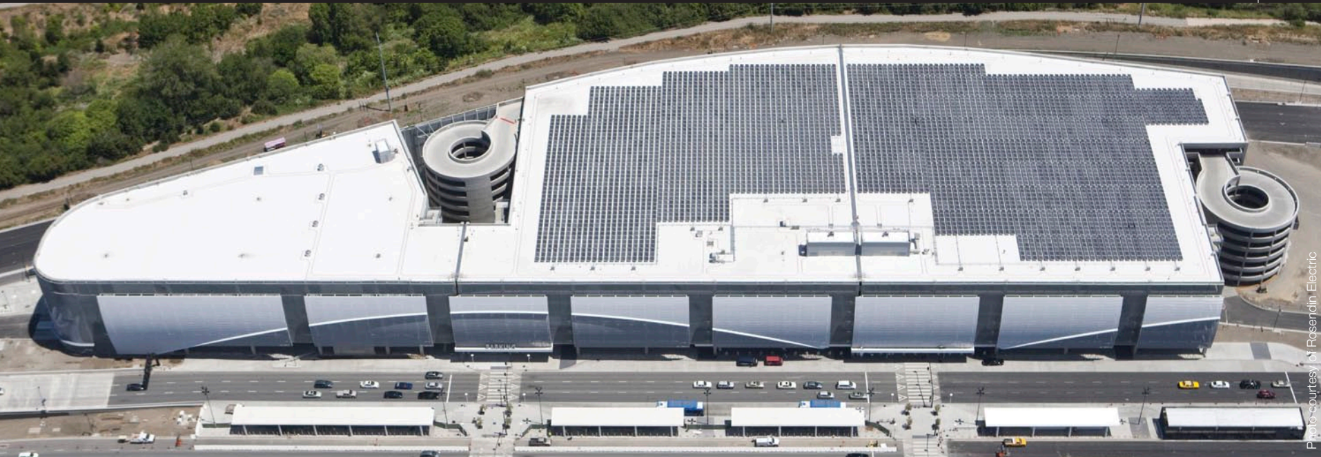
Rosendin Electric installed 4,680 solar panels covering 3.4 acres on the roof of the new CONRAC rental car facility at the San Jose Airport.
