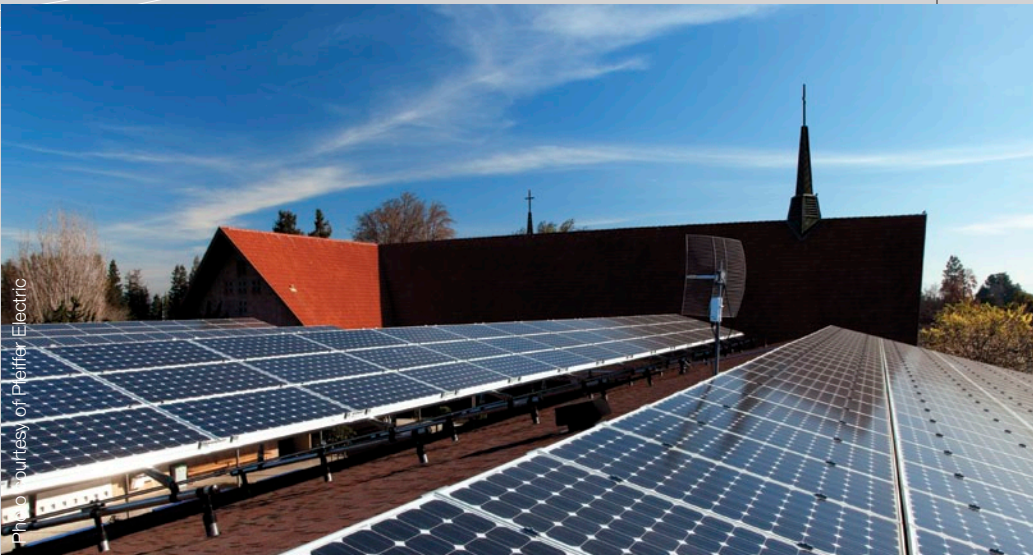
The Queen of Apostles Church and School is served by a 128 kilowatt solar system wired by Pfeiffer Electric.
