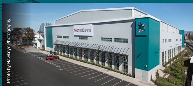
Sprig Electric Installs Electrical Infrastructure for Sharks Ice Arena Expansion in San Jose
