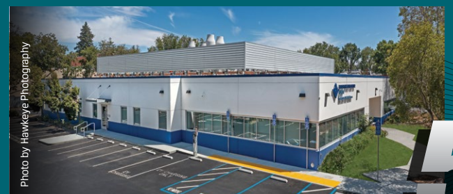
Yotta Electrical Services Installs Electrical Wiring In The New And Revamped TB And Refugee Clinic Of Santa Clara County
