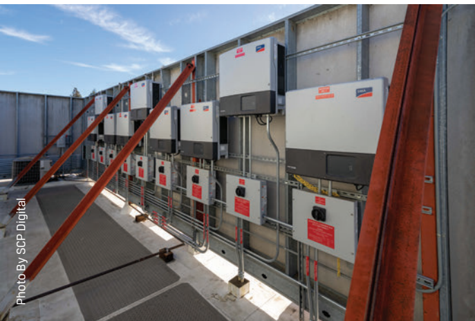
Pacific Ridge Electric installed nine inverters which convert energy into electricity for the building.
